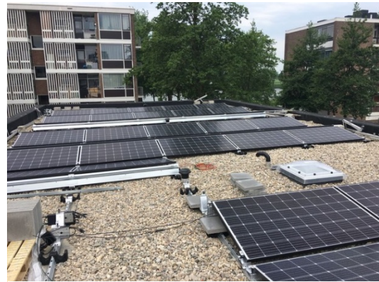
Figure 28: Renovation of flat roof; adding insulation and solar panels
