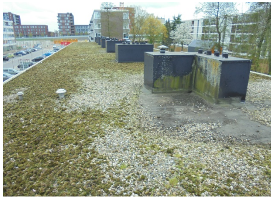
Figure 29: Flat roof, prior to renovation measures
